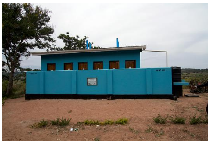
Sanzate Primary School's latrine after McGovern-Dole can help keep students, teachers, and administrators healthy.
